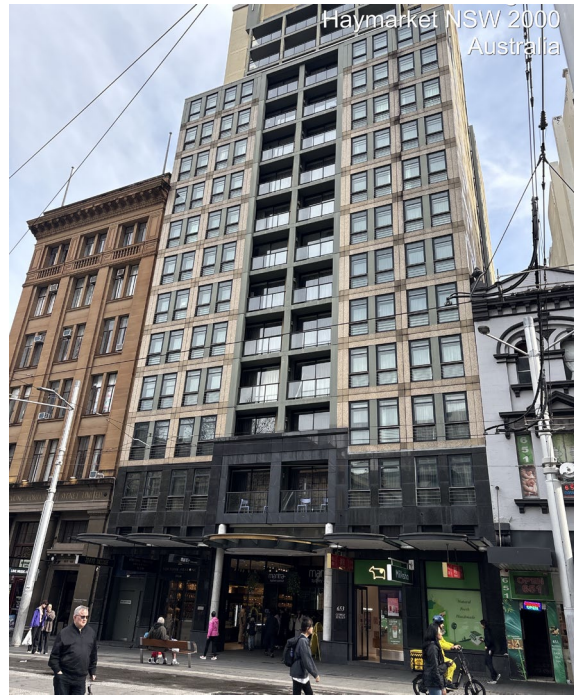
Figure 1: 653-659 George Street, Haymarket viewed from the north-west
